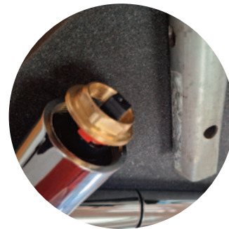
UNSCREW IN THE BRASS NUT
